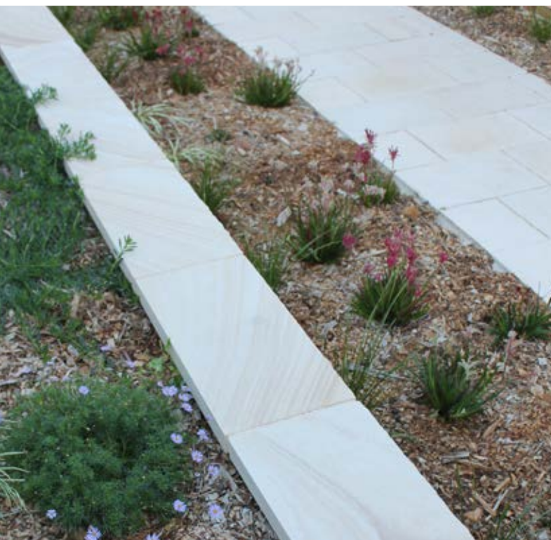
50mm Sawn Gosford Sandstone Capping, Rock-Faced on the front edges.
