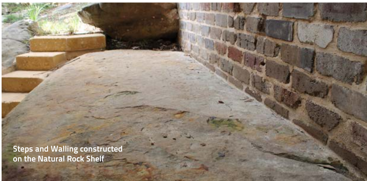
Reconstituted Sandstone Blocks used in the initial construction were utilised in these steps
